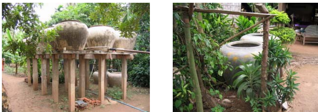
Figure 17: Water container put on higher level for gravity benefit to flow water in pipe
